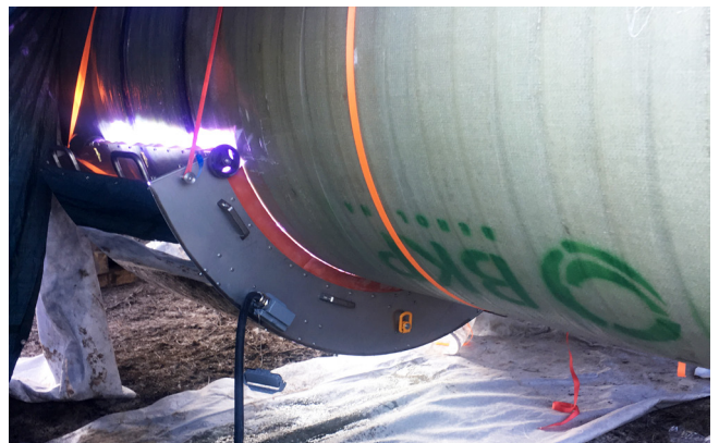
New UV technology for GRP weld protection, 2019
