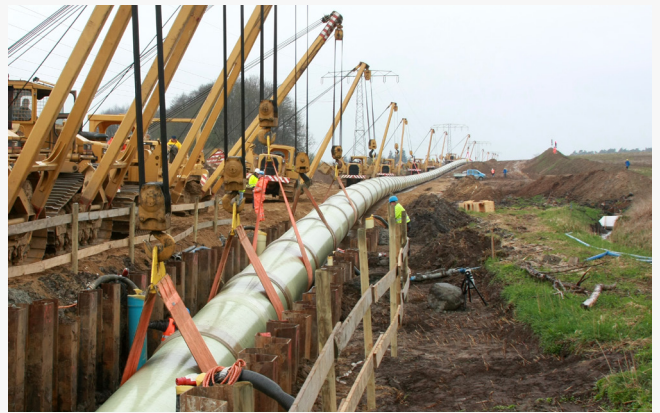
DN 1,400 GRP surface protection + GRP spacers
