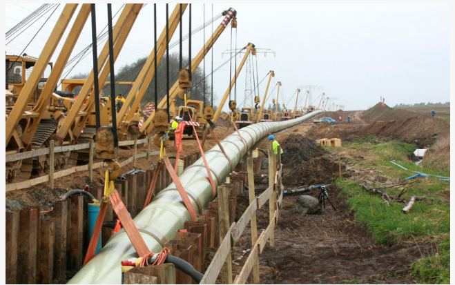
DN 1,400 GRP surface protection + GRP spacers
