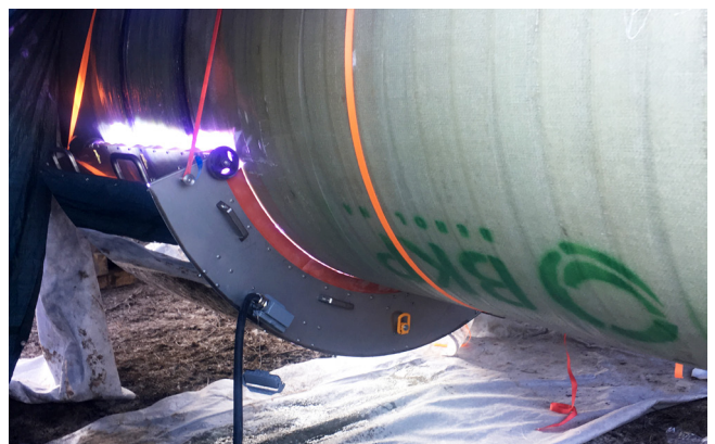
New UV technology for GRP weld protection, 2019
