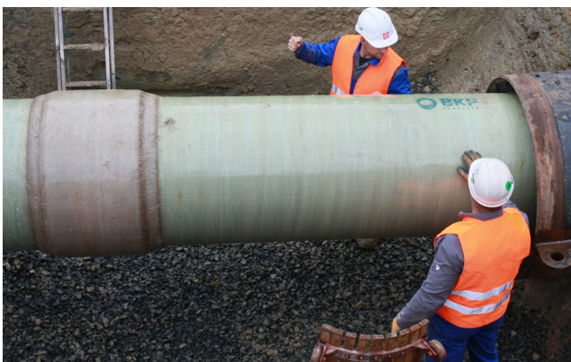
A tried-and-tested system: additional GRP spacers 2015
